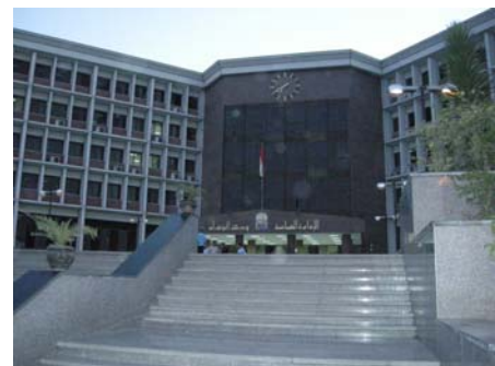
Hotel and Administrative building of the University of Assiut
